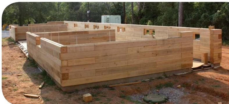
"Because we didn't want to use any heavy construction equipment," Frazier said, "we placed each of the 535 timbers by hand." And for the south wall, the team fabricated a glue-laminated beam onsite, which spans a 28-foot opening to accommodate the entry door and expansive windows.
