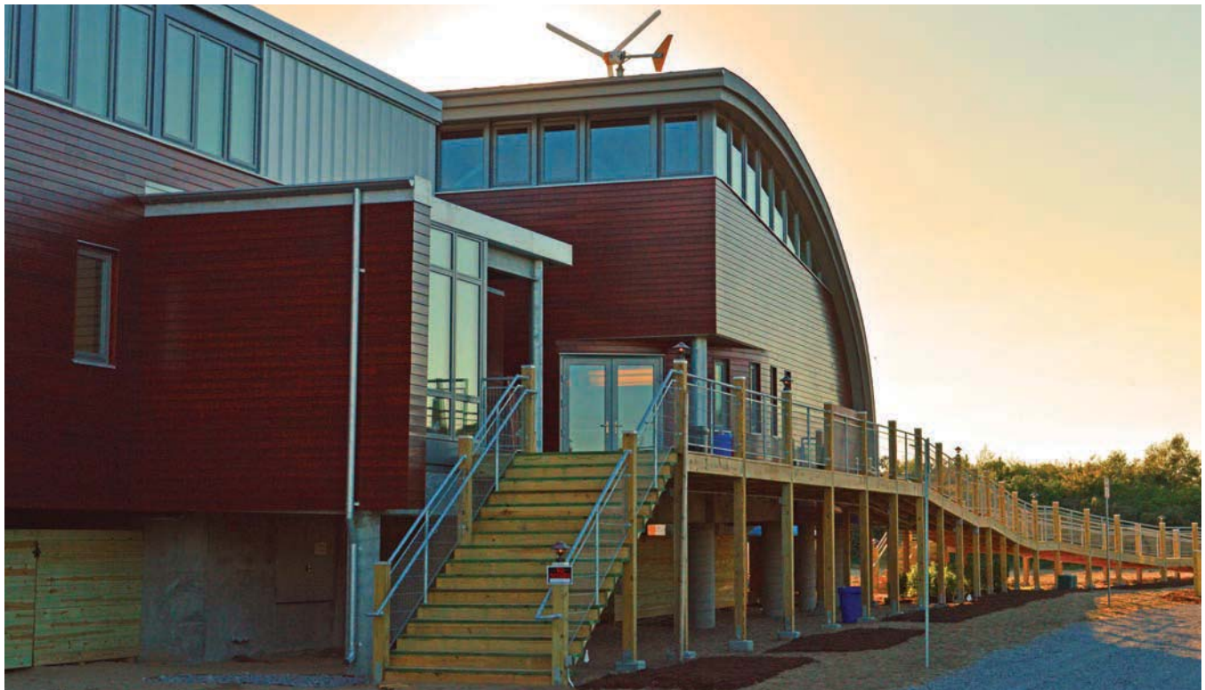
NATURALLY DURABLE: The Brock Environmental Center is 10,500 sq. ft., with 7,800 sq. ft. dressed in shiplap cypress siding. The facility is on pace to meet the requirements of the Living Building Challenge, a green building certification. (Photo by Chris Gorri)
